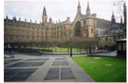
New Palace Yard.
