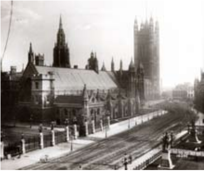
1890. Historic photographic view looking towards Old Palace Yard from Parliament Square showing the coordination of street furniture and landscape conceived by Sir Charles Barry, architect of the Palace of Westminster.
