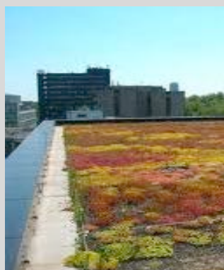
Extensive Green Roof - Use of a sedum mat only requires a 50mm build up and has limited structural implications
