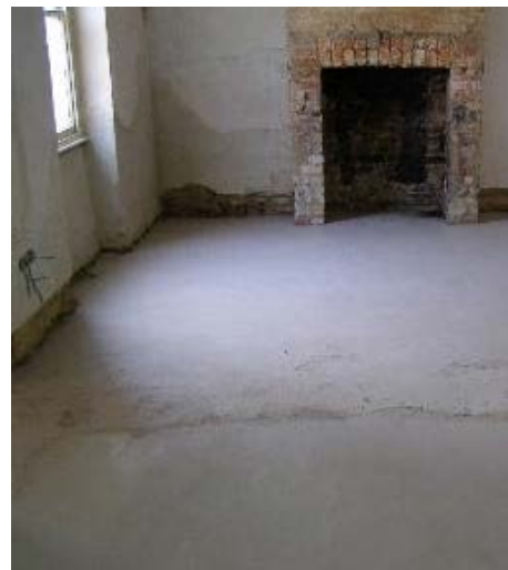
Concrete and screed floor
